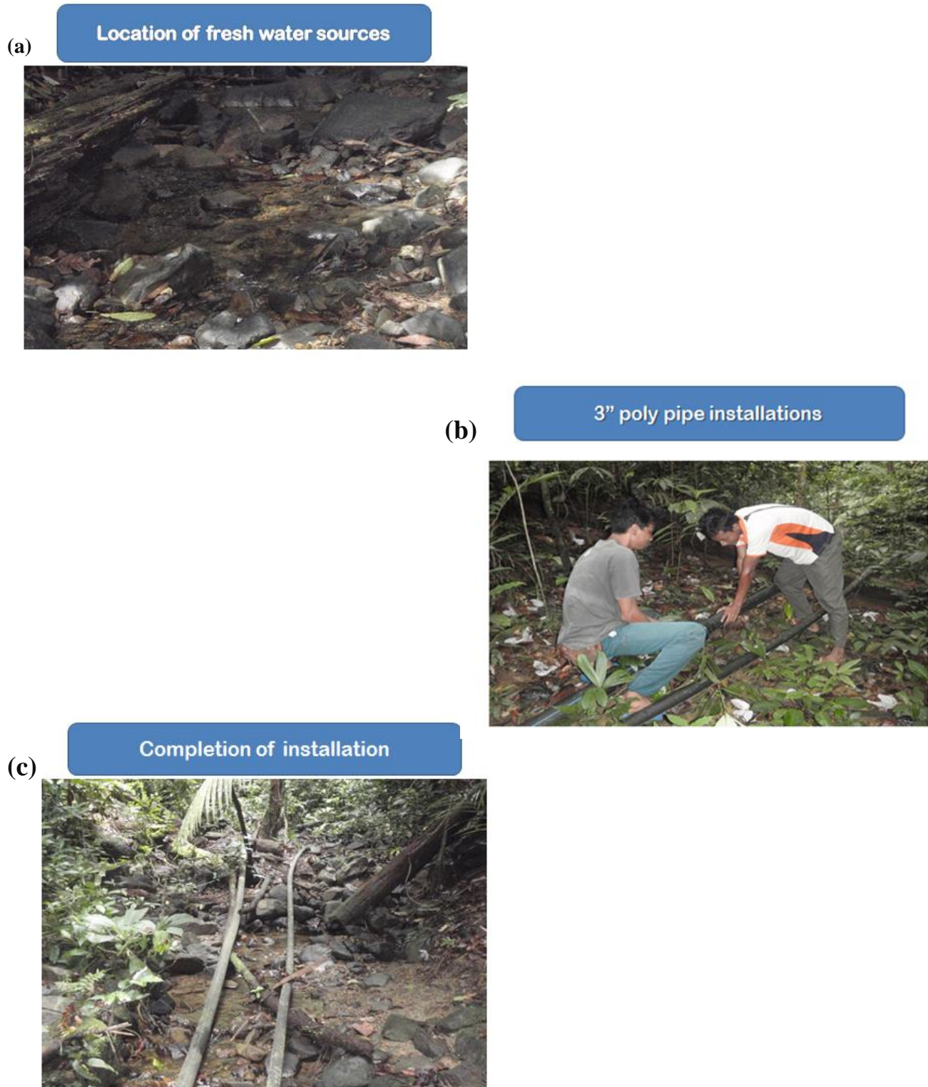
Fig. 10. The Community Water Catchment HCVF Project Installation
